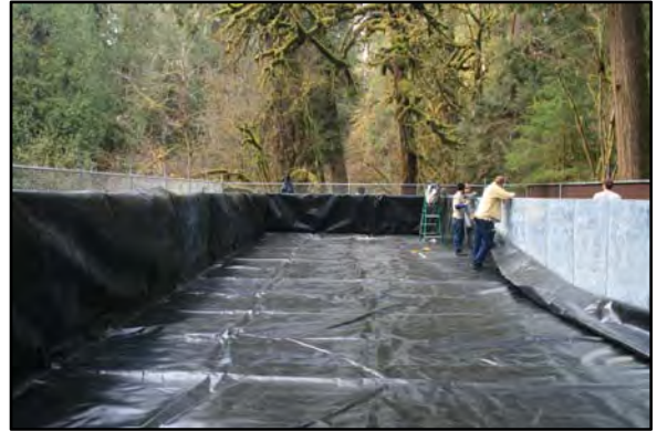
Acclimation Pond Construction
