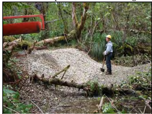
Bucket hauling gravel to Winter Arm Creek on Eel Lake.
